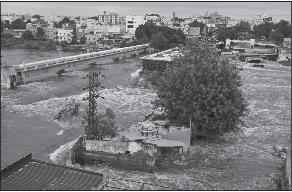
The Musi river flows in spate through the under-construction Moosarambagh bridge after heavy rainfall, in Hyderabad on Saturday
