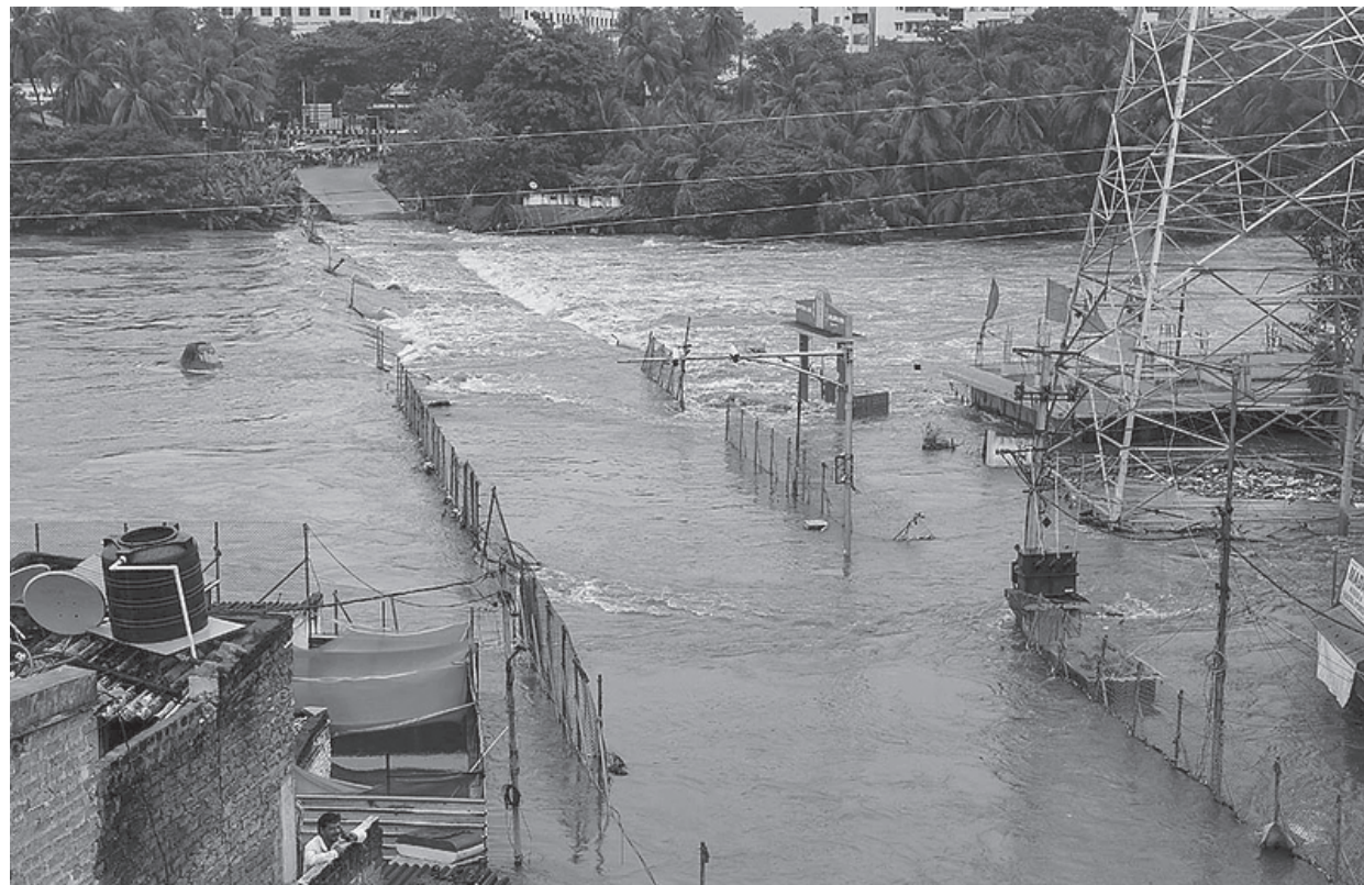
A flooded bridge over swollen Musi river following heavy rains, in Hyderabad on Saturday.
