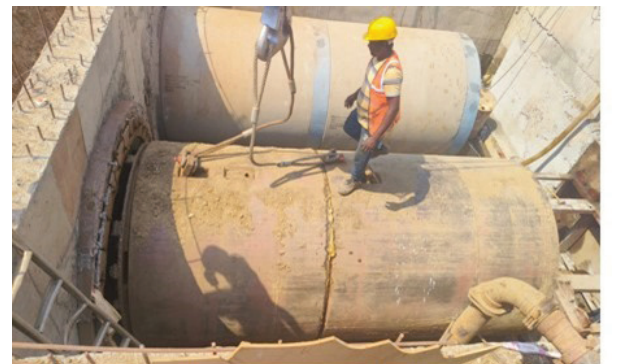
Micro-tunneling to augment discharge capacity
